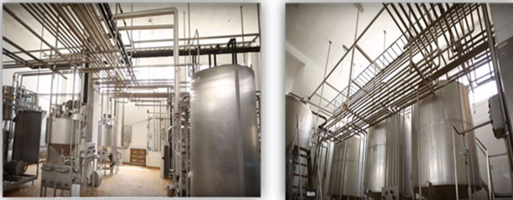
Figure 10: Machines of Al-Safa dairy factory.
